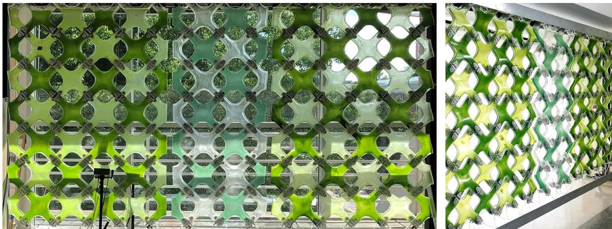
Figure 12: Final assembled microalgae façade with five different strains of microalgae.
