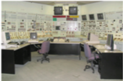
PLC Pickering Unit 1-4 Simulator
